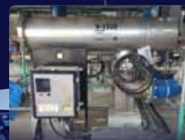
COOLING TOWER Chemical-Singapore
